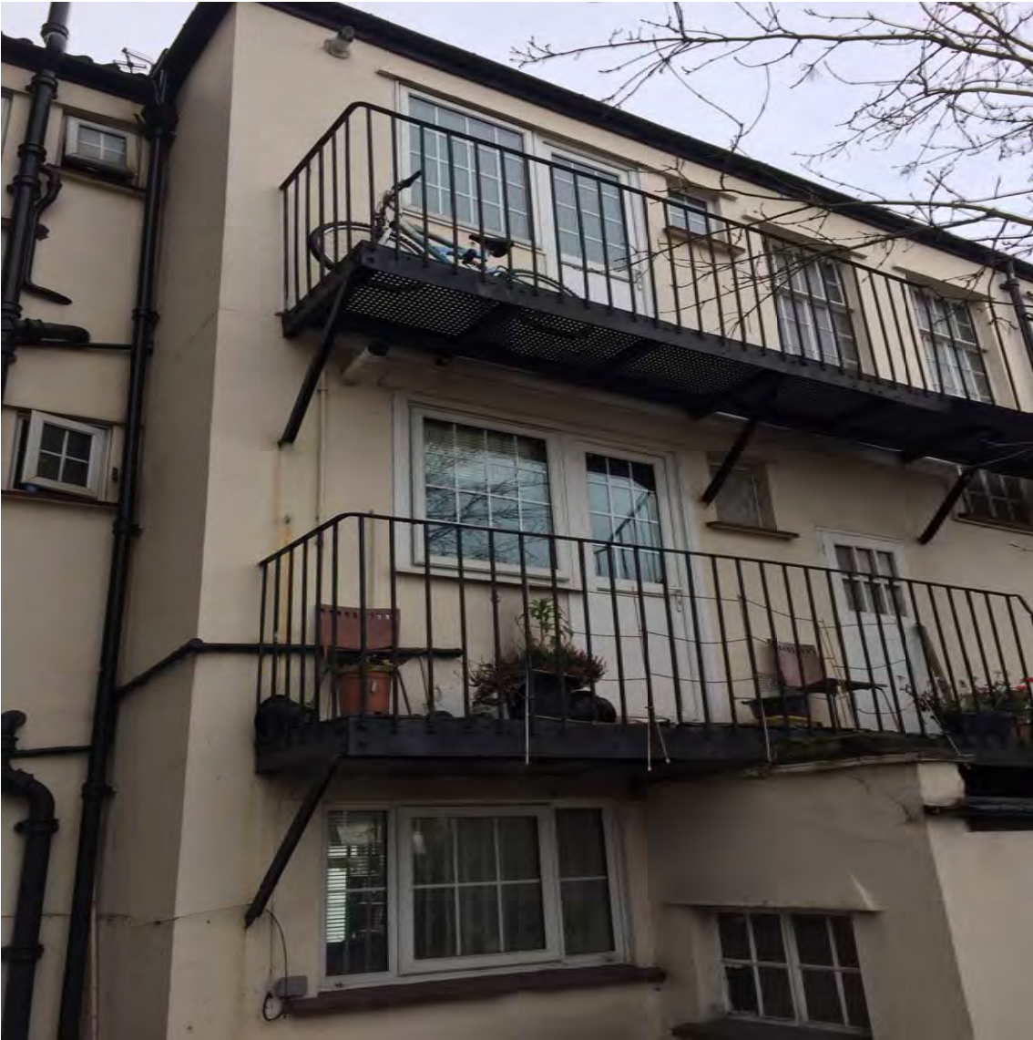
Rear elevation of No. 39 Lowlands Road
